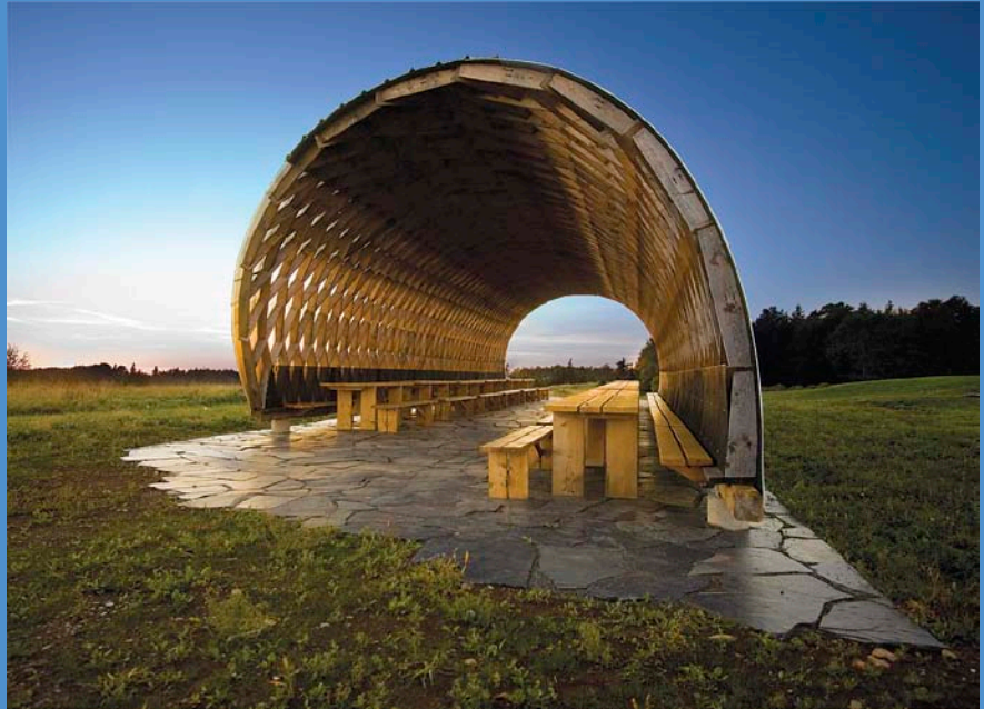
Lamella arch serves as dining pavilion at Ross Creek Centre for the Arts in Canning, Nova Scotia
